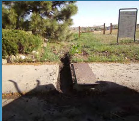
Sidewalk Chase Silt Removal
