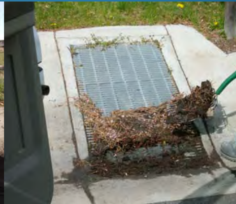
Grate Cleaning Ponds & Inlets
