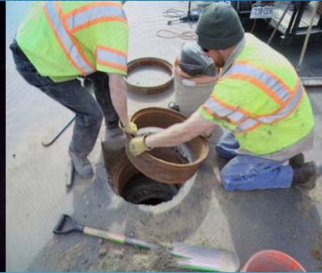
Raising Buried Manholes in Four Square Mile Area
