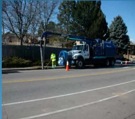
Inlet/Vault Cleaning
