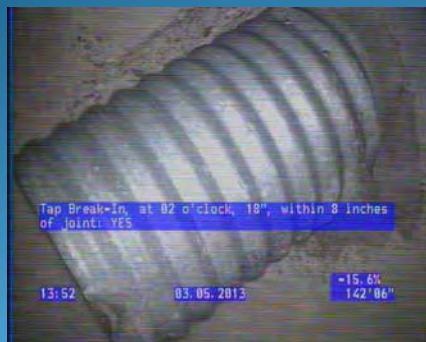
Protruding Tap-in & No Manhole
