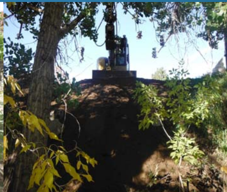
Filling & Compacting Slope
