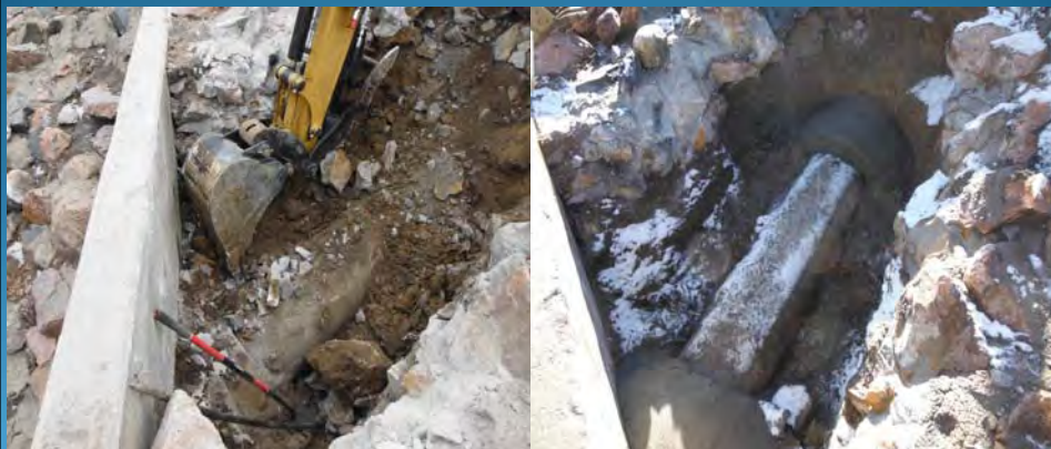
Excavating to Expose Pipe
