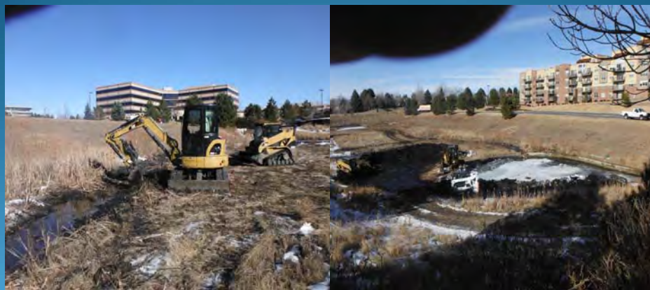
Cleaning Rock-lined Channel
