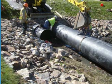
Installing Lining
