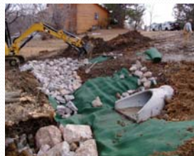
FLARED END SECTION REPLACEMENT & BANK REPAIR
