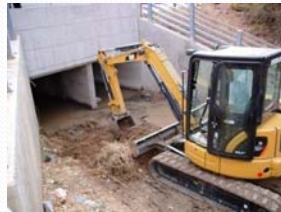
CULVERT CLEAN OUT
