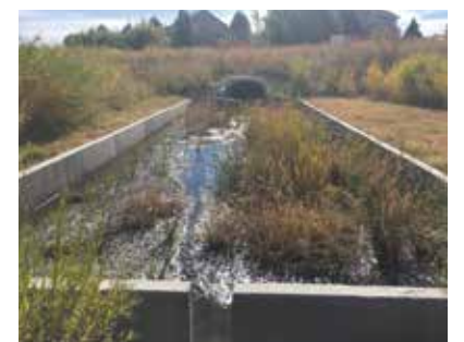
Outfall structure w/forebay
