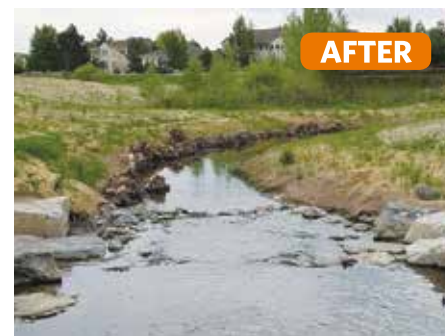
A heavily eroded reach of Piney Creek reclaimed with channel grade control and a bank protection test section using tree root wads.
