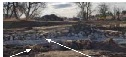
Root wads line the bank, reinforced by hard armoring
