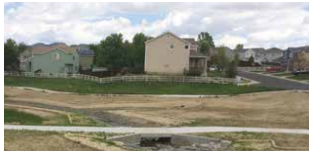
Redefinition of the Piney Creek Reach 7 channel west of Liverpool Street, with stabilized banks decreasing sediment transport downstream to Cherry Creek
