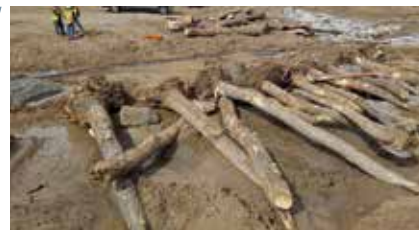
Tree root wads ready for placement along the bank
