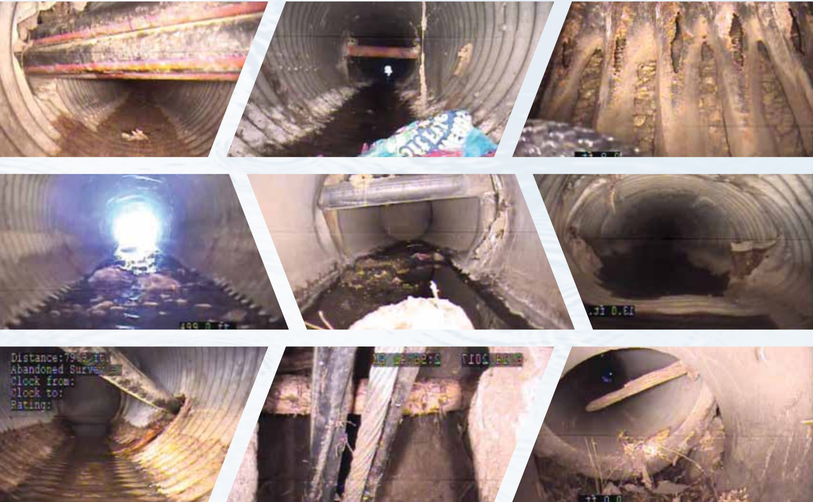
Damaged corrugated metal pipe discovered initially during 2017 CCTV inspections that will result in multiple pipe-lining projects or full pipe replacement projects.
