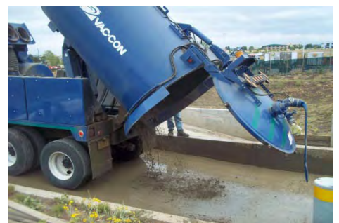
Jet-truck disposal of removed sediment & wastes
