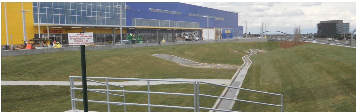
The extended detention basin water quality treatment facility at the IKEA Centennial store
