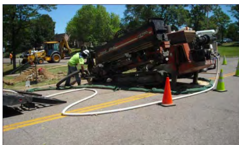
Typical directional boring for dry utility work
