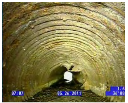
Corrugated metal culvert as shown in pipe video
