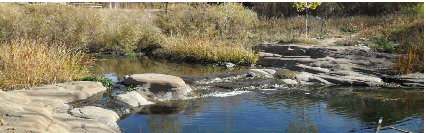
Sculpted drop grade control structure in Fox Hill Park on West Toll Gate Creek
