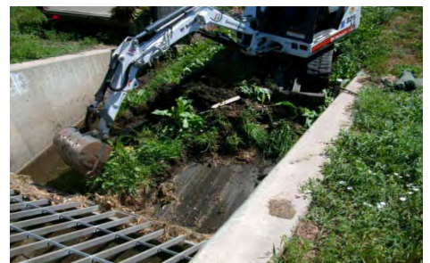
Removing vegetation & debris from infrastructure
