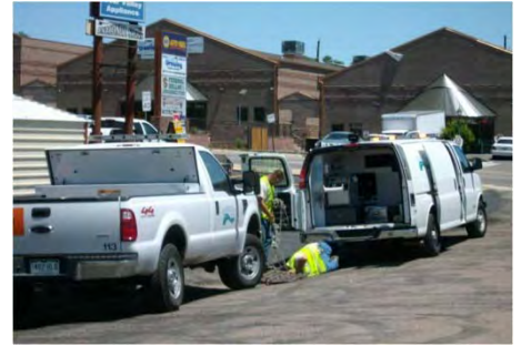
Crew videoing storm sewer pipe for inventory
