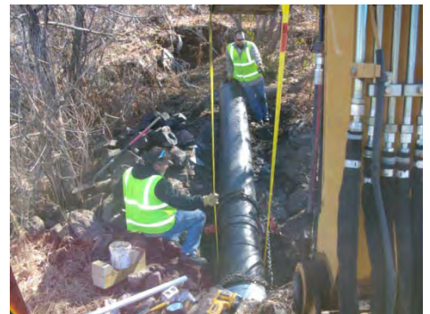
Maintenance Crew slip lining the culvert segment
