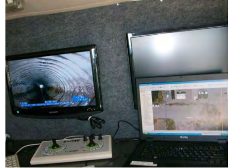
Inside the Pipe Video System Van
