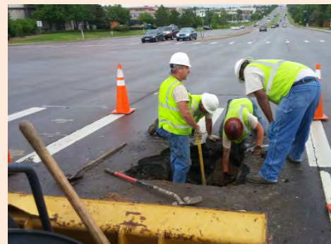
Putting final touches on concrete replacement
