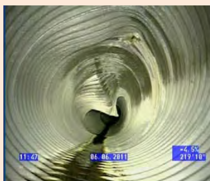
Damaged pipe at Mineral Ave/Vincennes Way
