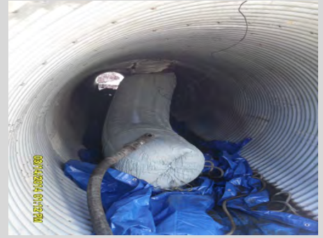
Resin tube is pressurized to cure 'new' pipe
