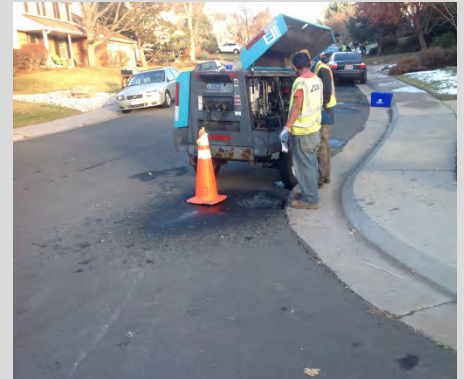
Investigating a hydraulic fluid spill from a residential generator, requiring source elimination and cleanup
