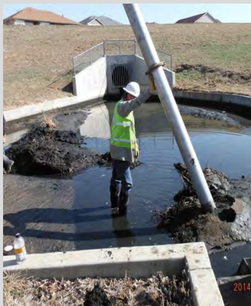
Cleaning sediment collected in detention pond forebay
