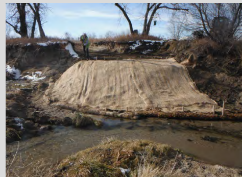
Removing an illegal bridge obstruction in the Piney Creek floodplain to resolve a permit violation; a designed pedestrian bridge will be built as part of a future CIP project
