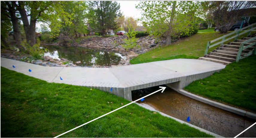
A new low water crossing replaced an older pedestrian bridge, and a new box culvert crossing replaced a break-away fence to ensure adequate flood conveyance
