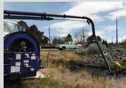
Cleaning outfalls & inlets with the Vactor® truck
