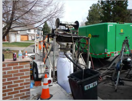
Cured-in-Place (CIPP) pipe technology onsite
