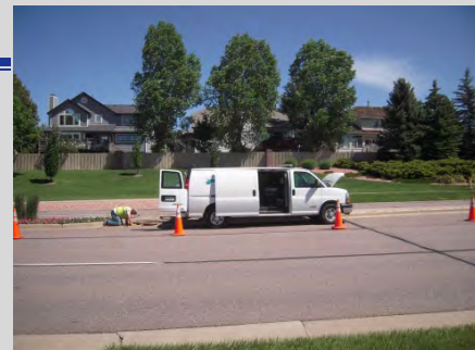
Camera Van televising storm sewer pipe system
