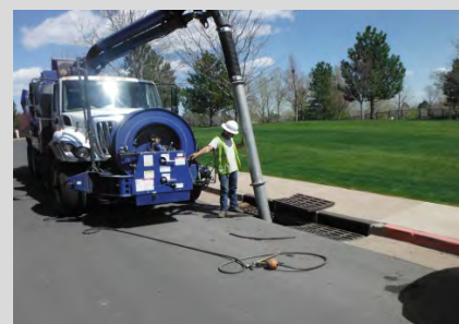
Cleaning outfalls & inlets with the Vactor® truck
