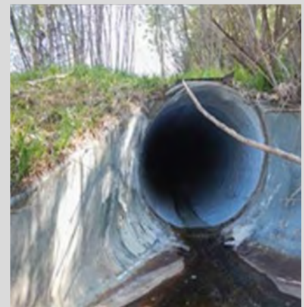
A rehabilitated corrugated metal pipe outfall
