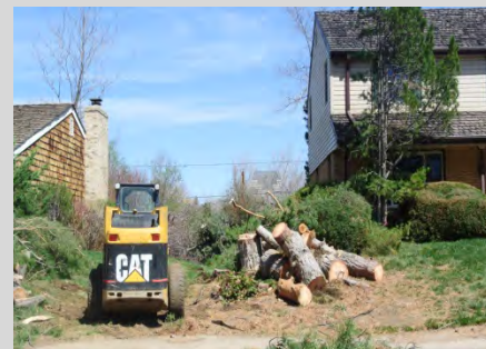
Prepping an easement for a CIP construction project
