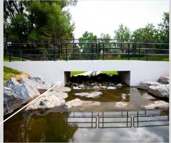
A new low water crossing replaced an older pedestrian bridge, and a new box culvert crossing replaced a break-away fence to ensure adequate flood conveyance
