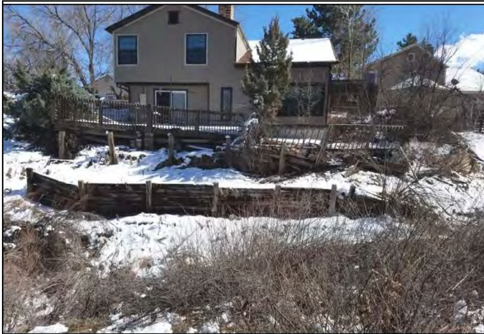
Figure 1. View of 3 failing timber retaining walls on the right (east) bank of West Spring Creek at 8019 S Niagara Way. The lower wall is being undermined by the creek.
