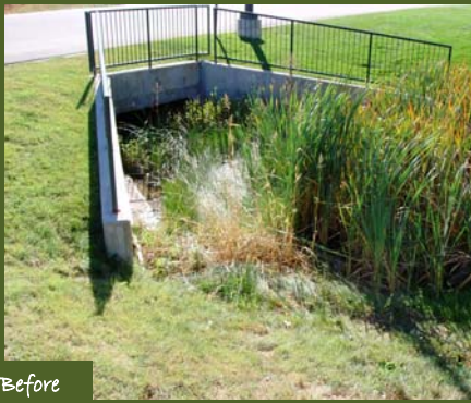
Briarwood/Potomac culvert cleanout project
