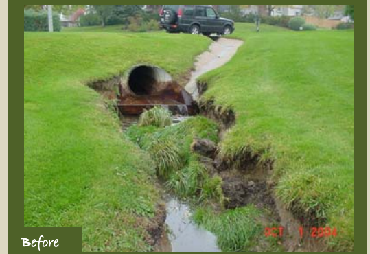
Willow Creek conveyance system remedial project
