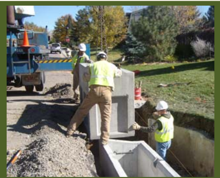
Easter/Verbena Infrastructure Project
