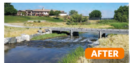
Reclaimed channel & golf cart low water crossing
