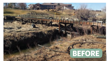
Cherry Creek channel and golf cart bridge
