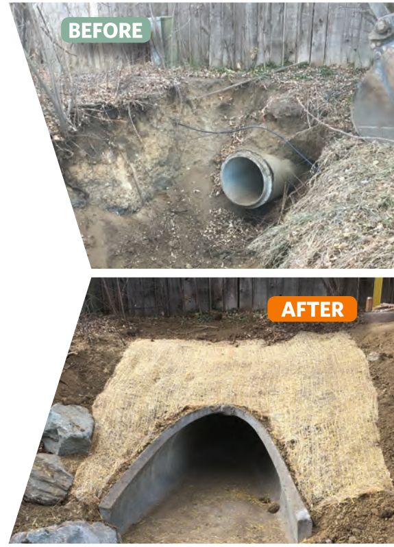
RIGHT: A routine pipe inspection identified an outfall into Big Dry Creek in need of repair to minimize erosion of the channel banks. BELOW: East Toll Gate Creek at Dove Hill subdivision experienced sediment buildup at the Progress Street roadway culvert (1), causing local flooding. Initial work consisted of vegetation management (2 and 3), followed by a maintenance project to re-establish a low flow channel through the culvert (4) to provide unobstructed conveyance for the storm runoff events.
