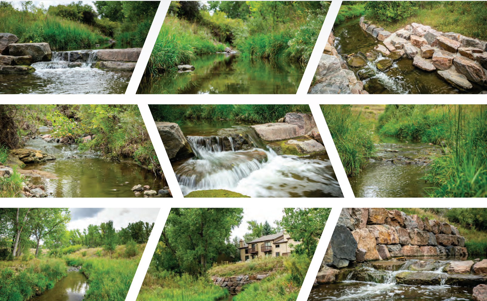
The completed Willow Creek, Quebec to Dry Creek Channel Improvements project included stream stabilization, bank protection, and a grade control drop structure to protect a sanitary sewer line.
