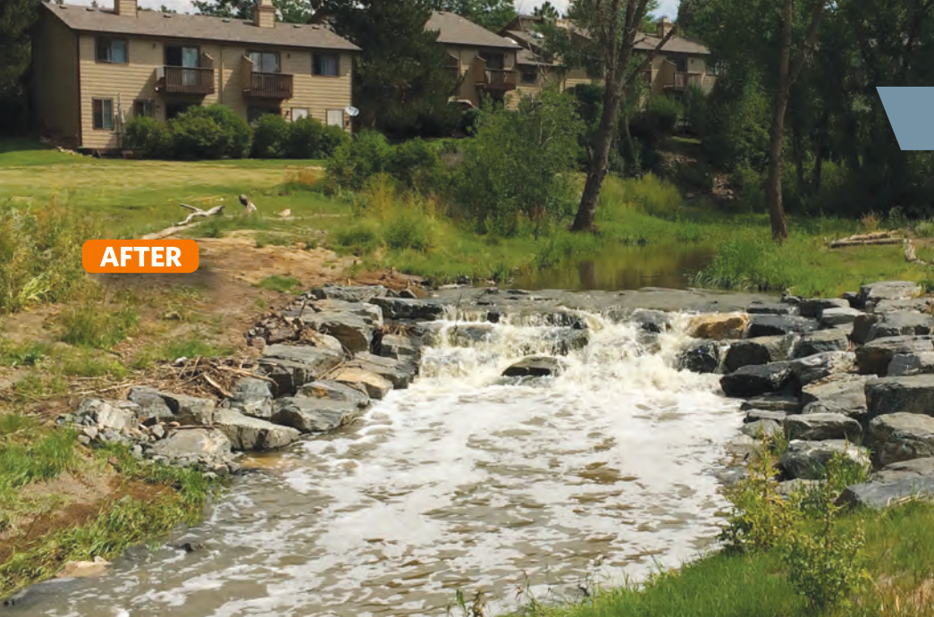
Reclamation of Willow Creek downstream of Quebec, resulting in a stable channel that can carry base flows and flood flows without erosion and transport of sediment.
