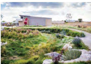
A Green Living wall (above) and vegetated swales (below) are two of the infiltration approaches demonstrated, with a path through the demo site to guide visitors to features that promote lot-level control measures.
