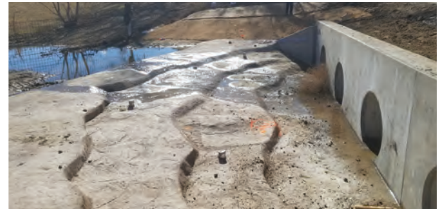
Reclamation of Willow Creek downstream of Quebec, resulting in a stable channel that can carry base flows and flood flows without erosion and transport of sediment.
