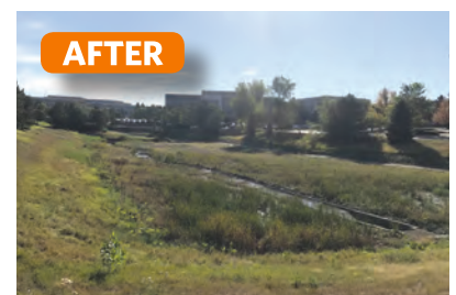
At the Panorama Pond, a formalized low flow trickle channel improves conveyance of flows, and a functioning outlet structure will detain an appropriate volume of water and allow for the collection of sediment and trash.
