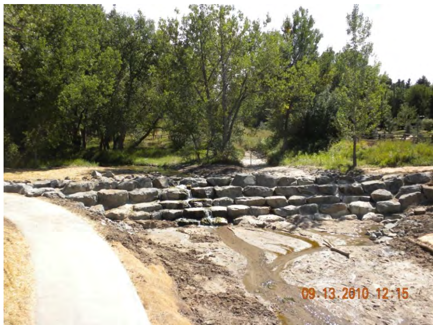
LOOKING UPSTREAM AT BOULDER DROP STRUCTURE
