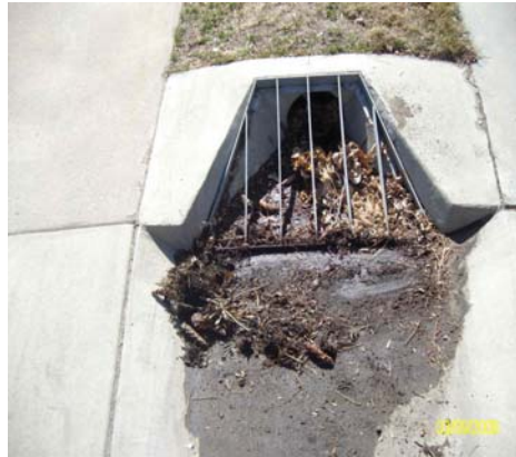
Pipe and Grate Cleaning
