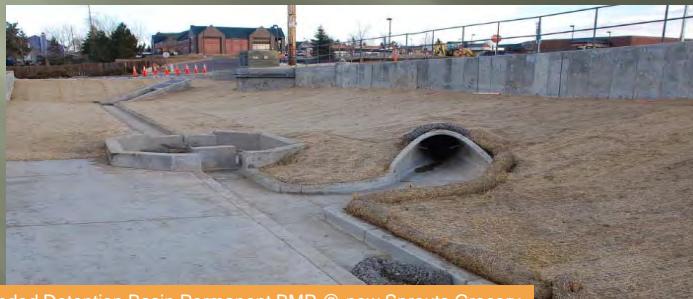
Extended Detention Basin Permanent BMP @ new Sprouts Grocery
