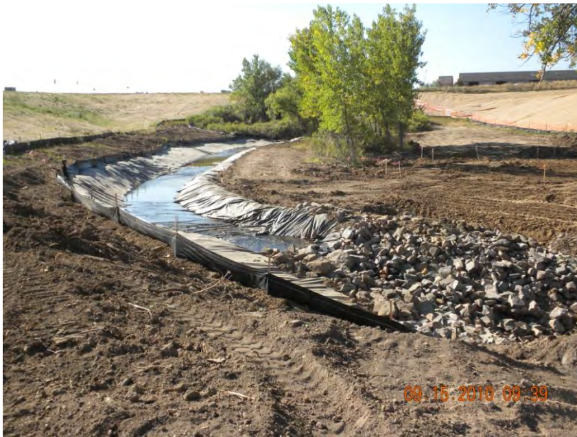
DIVERSION AROUND DROP STRUCTURE
